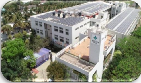
Manufacturing facility at Chikkaballapur
