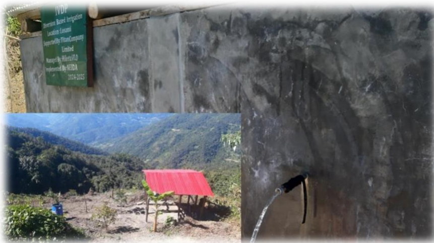
Figure 11: Diversion based irrigation facility at Losami
