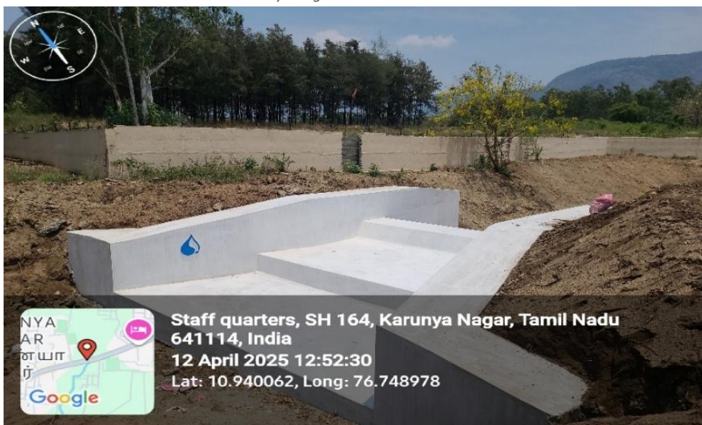
Check dam #5 after reconstruction and desilting
