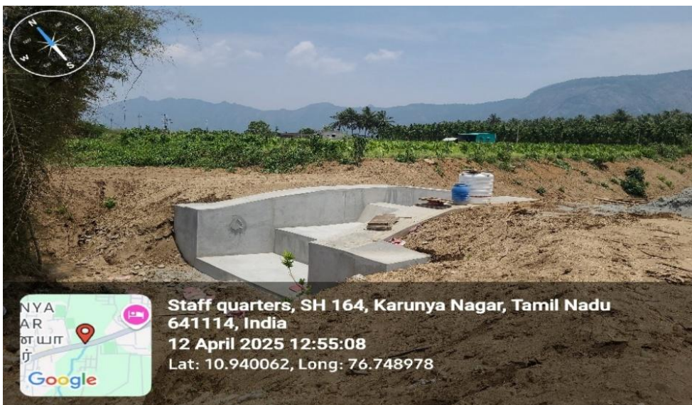
Check dam #6 after reconstruction and desilting
