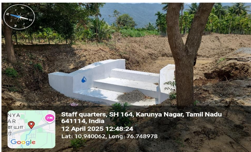
Check dam #3 after reconstruction and desilting
