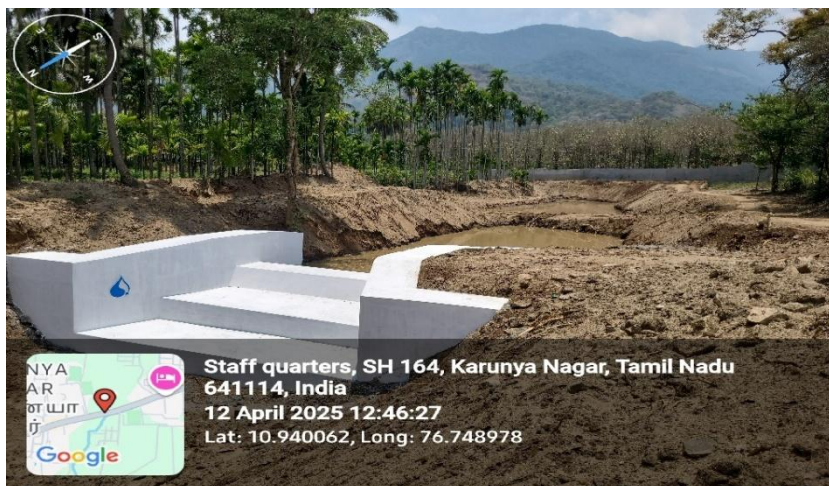
Reconstructed Check dam #2 and desilting is complete
