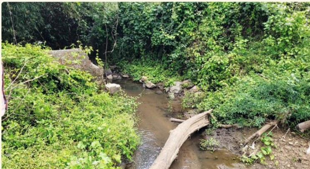
Check Dam #5 — only wing walls and no weir wall at baseline.
