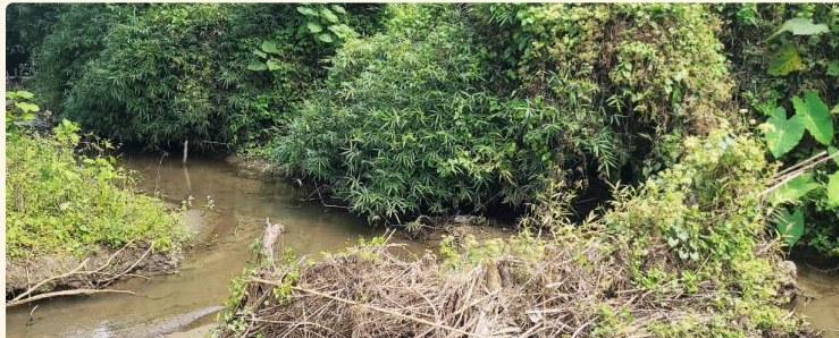
Check Dam #2 — only wing walls and no weir wall at baseline.
