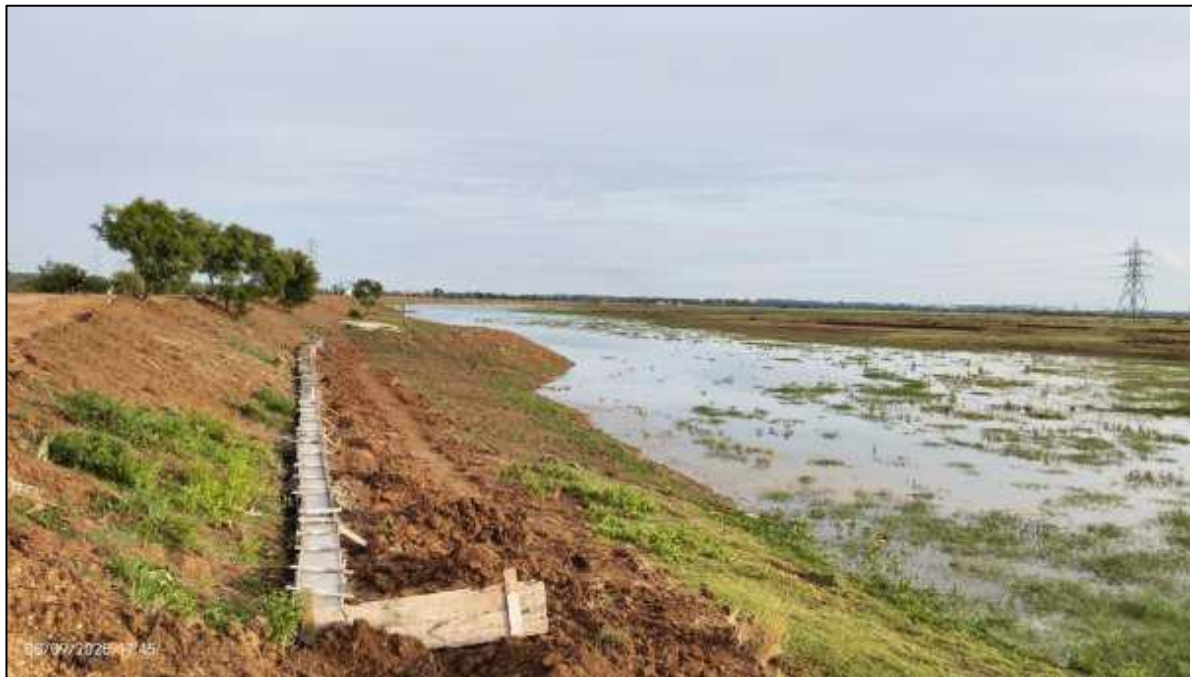
Figure 2.5 a): Toe wall constructed at the base of the Bund
