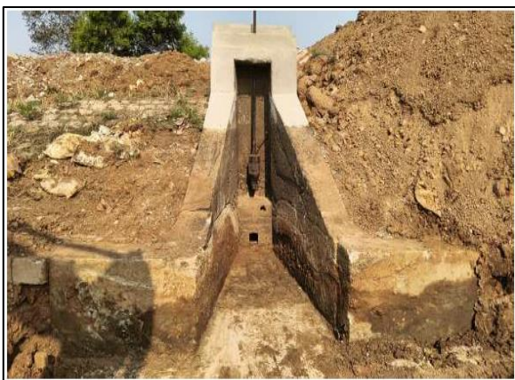
Sluice gate before restoration
