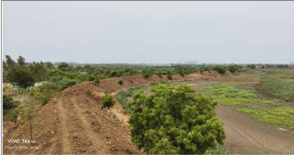
Figure 2.4 a): Bund formed using excavated soil
