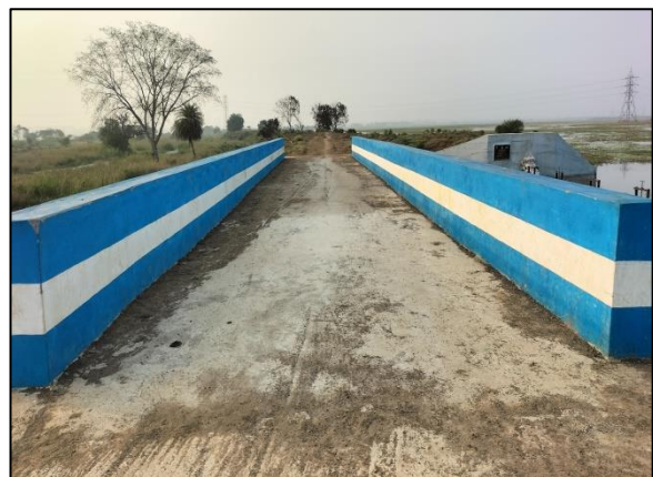
Walkway after restoration
