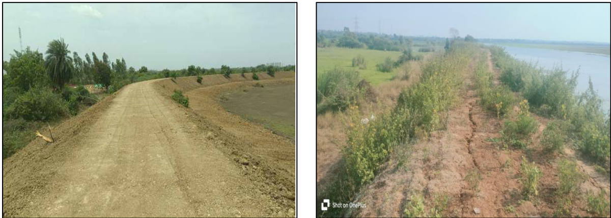
Figure 4.3: Photographs of the bund after restoration and its present status
