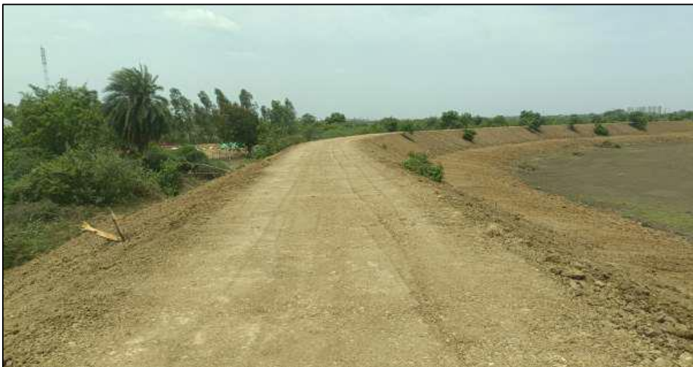
Figure 2.4 c): Bund after restoration
