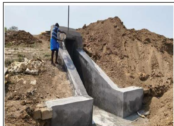
Sluice gate after restoration
