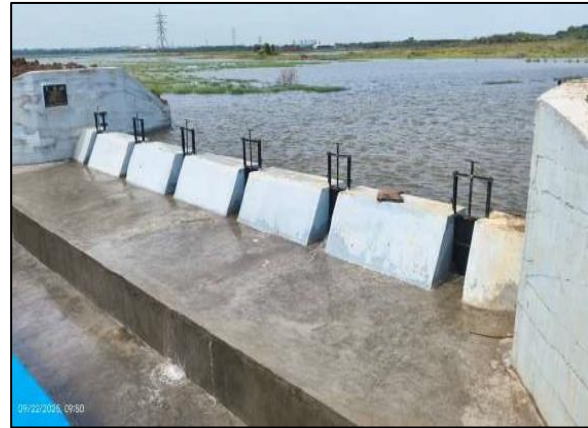
Weir after restoration
