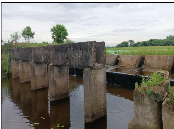
Walkway before restoration
