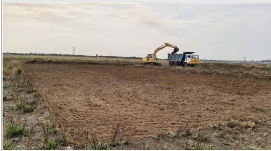
2.2 b): Drone image of the lake during restoration
