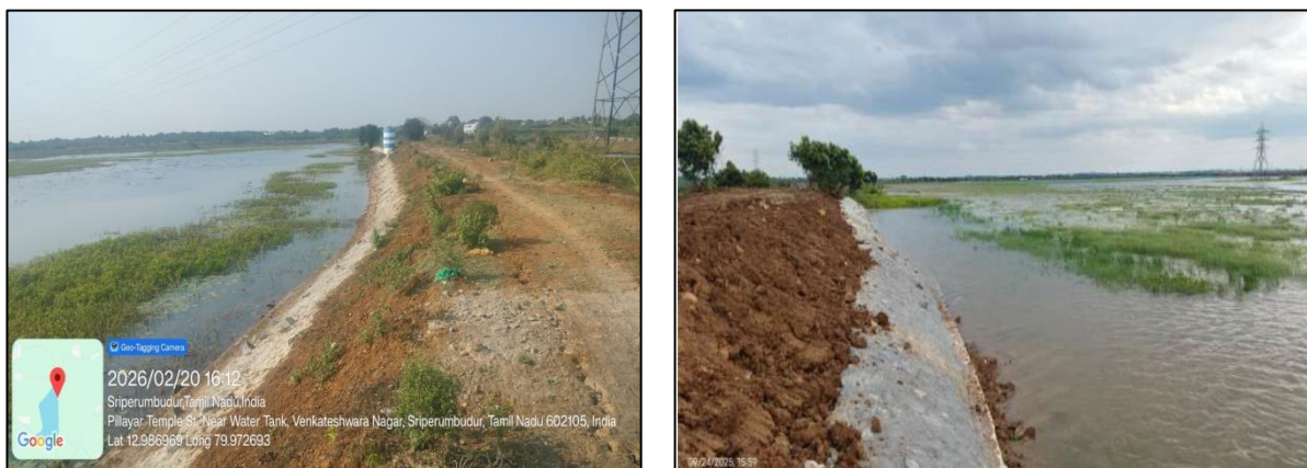
Figure 2.5 b): Stone pitching done near the sluice gates and weir
