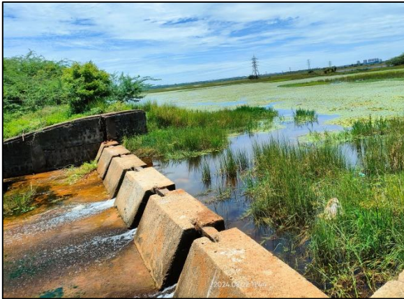
Weir before restoration
