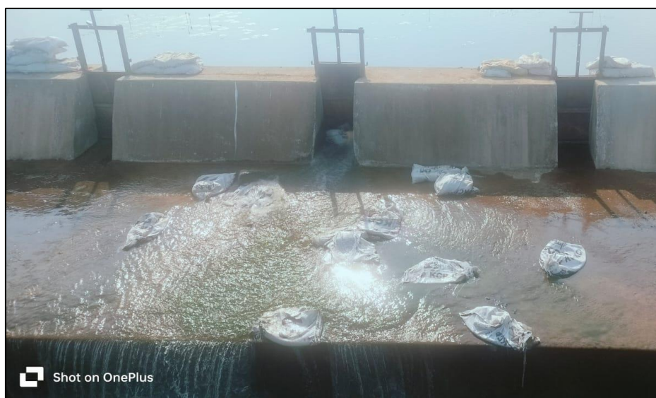
Figure 4.4: Photograph showing use of sand filled bags to regulate water flow
