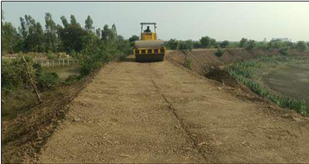
Figure 2.4 b): Consolidation of the Bund in progress
