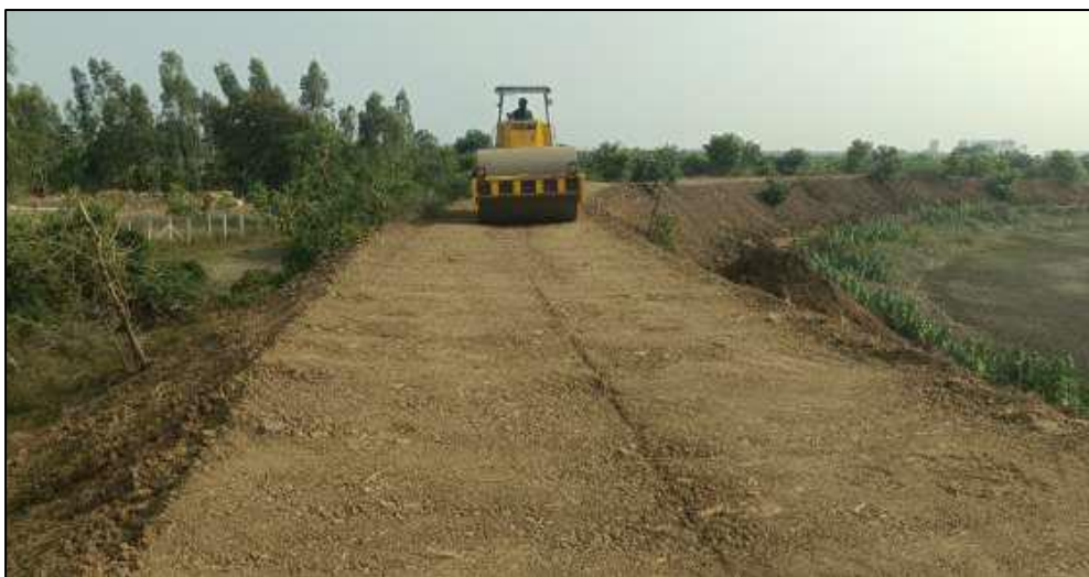
Figure 2.4 c): Consolidation of the Bund in progress
