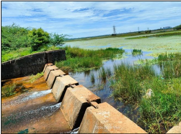
Weir before restoration
