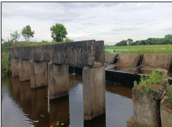
Walkway before restoration
