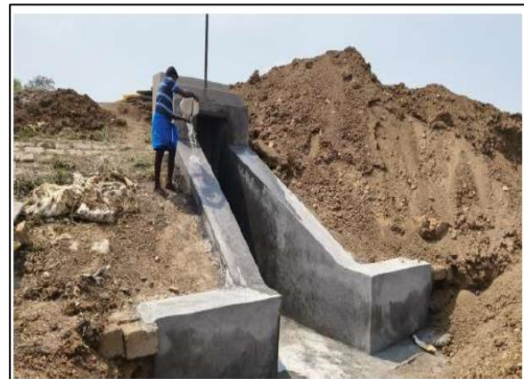
Sluice gate after restoration
