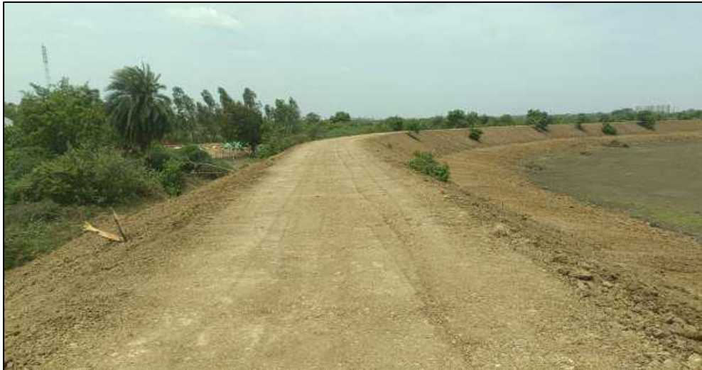
Figure 2.4 d): Bund after restoration
