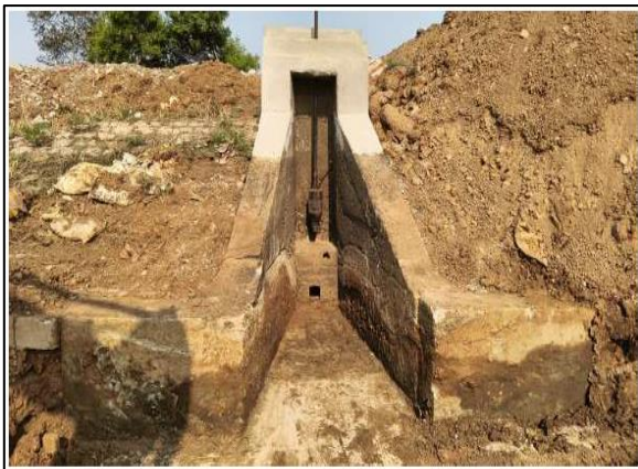
Sluice gate before restoration
