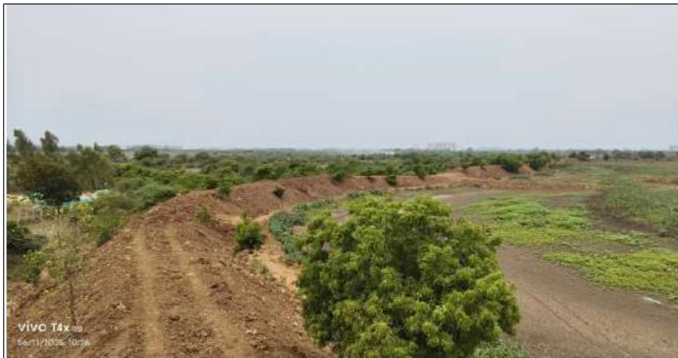
Figure 2.4 b): Post restoration Bund formed using excavated soil
