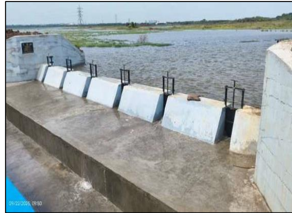
Weir after restoration
