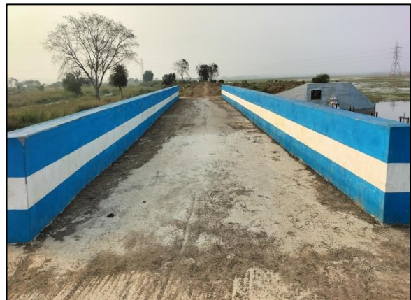
Walkway after restoration
