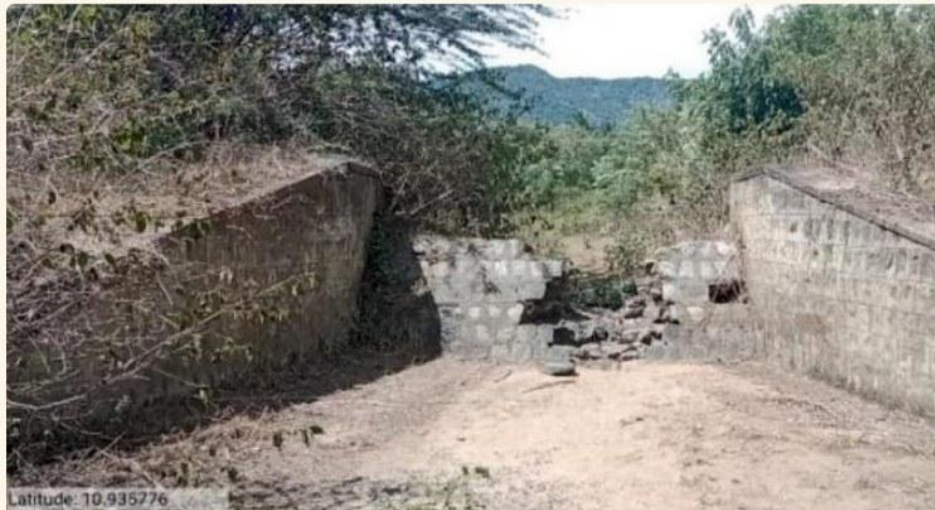
Check Dam #6 — only wing walls and severe damage to weir wall at baseline.
