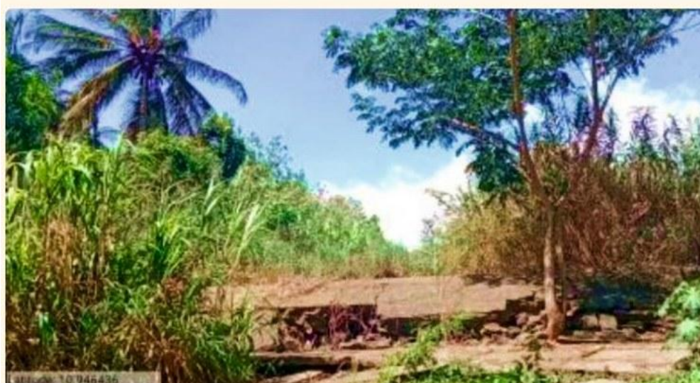
Check Dam #7 — no wing walls and no weir wall at baseline; the largest silt removal on the corridor.
