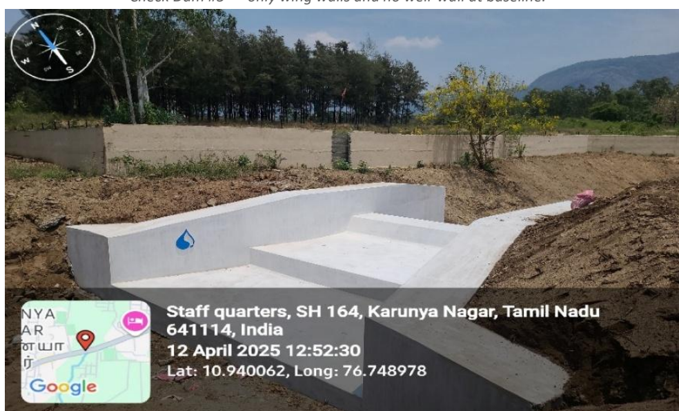
Check dam #5 after reconstruction and desilting
