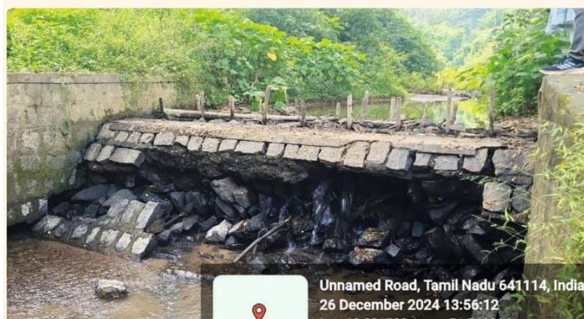
Check Dam #3 — severe silt accumulation, cracks and seepage in the weir; almost inaccessible at baseline.
