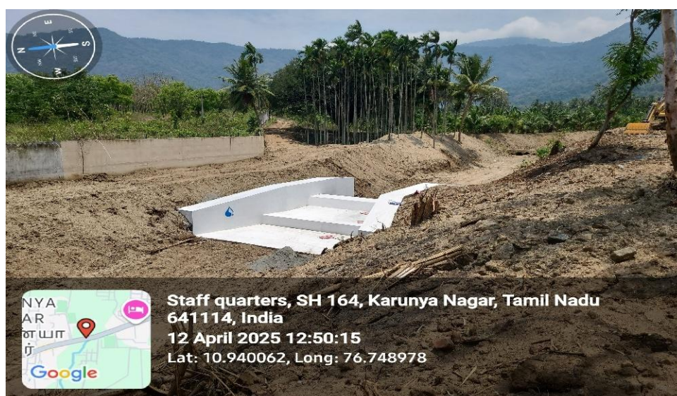
Check Dam #4 — only wing walls and no weir wall at baseline.
