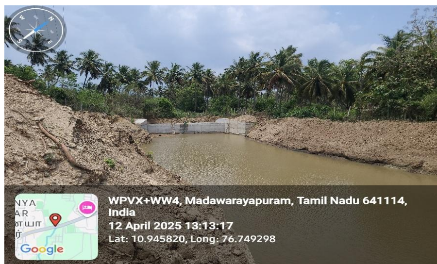
Check Dam #7 — no wing walls and no weir wall at baseline; the largest silt removal on the corridor.
