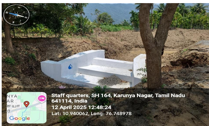
Check dam #3 after reconstruction and desilting
