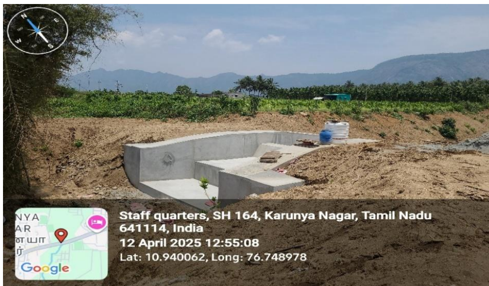
Check dam #6 after reconstruction and desilting
