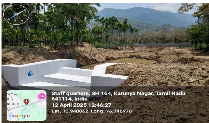
Reconstructed Check dam #2 and desilting is complete
